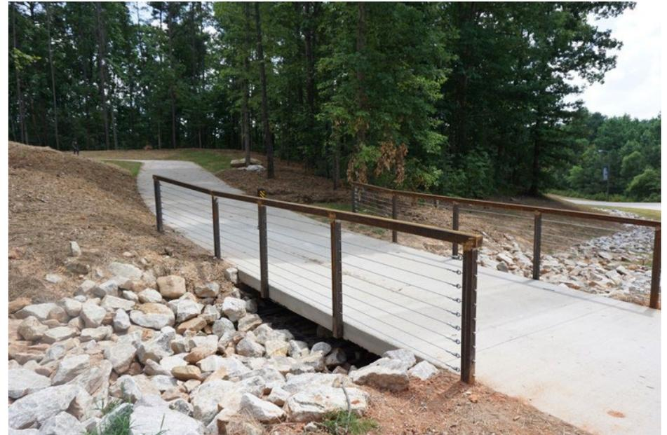
*Examples of the use of structural slabs in a trail.*
