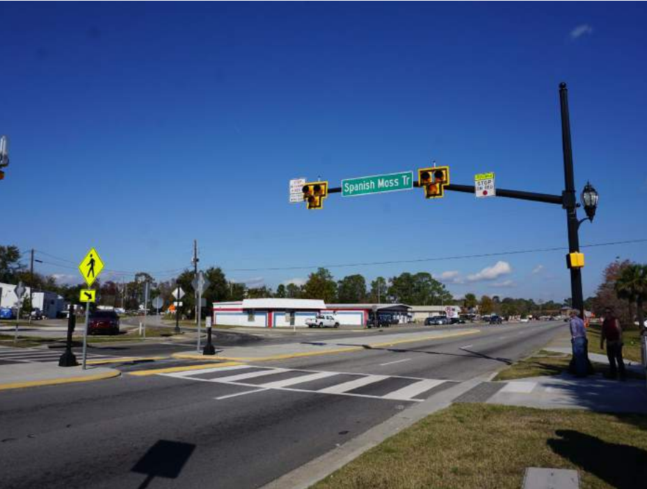
Example of a trail crossing with a pedestrian hybrid beacon (a.k.a. “HAWK” signal)
