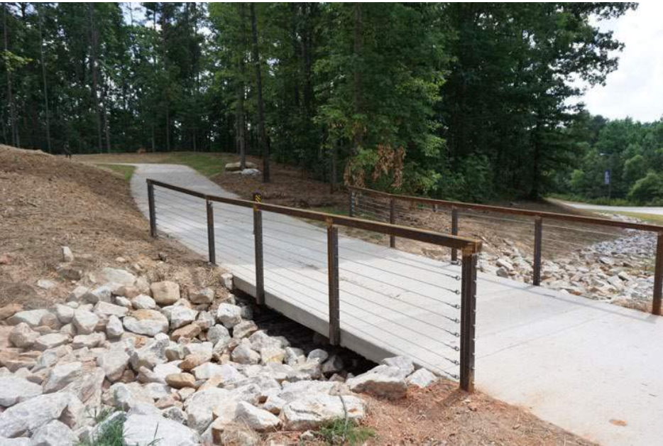
Examples of the use of structural slabs in a trail.
