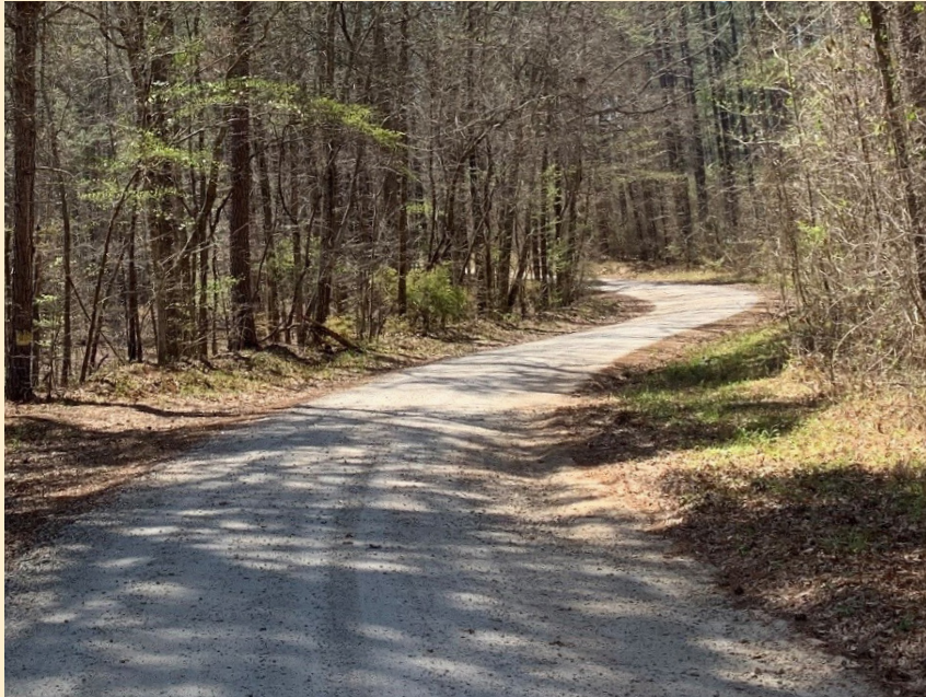
Example of crusher run used to create a road.
